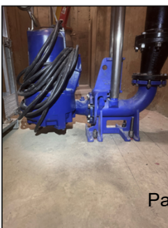
Inside Wet Well – Sump Pump
